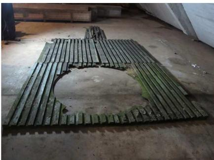
**T86 Roof Decking Laid Out after Removal**
